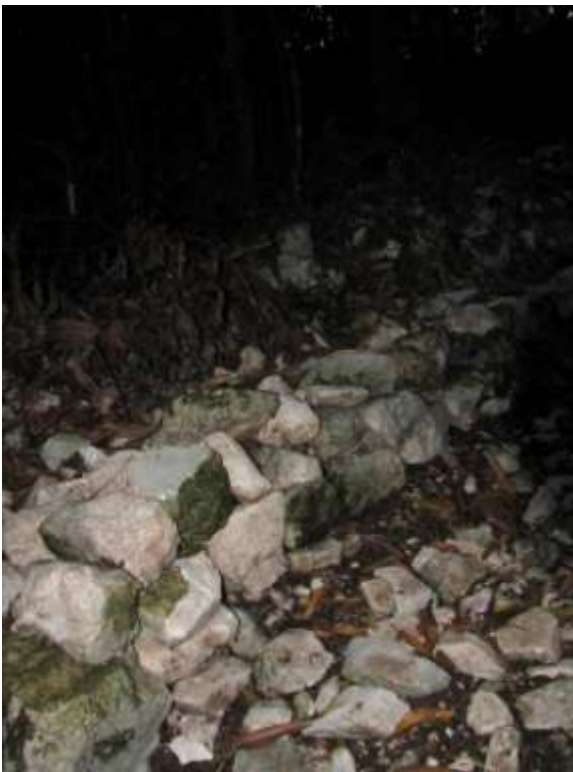
Figure 77: Dry stone wall
